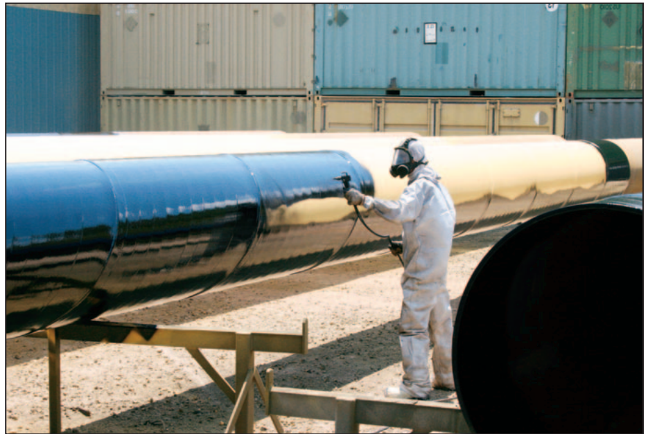
Application of specialized coating.
