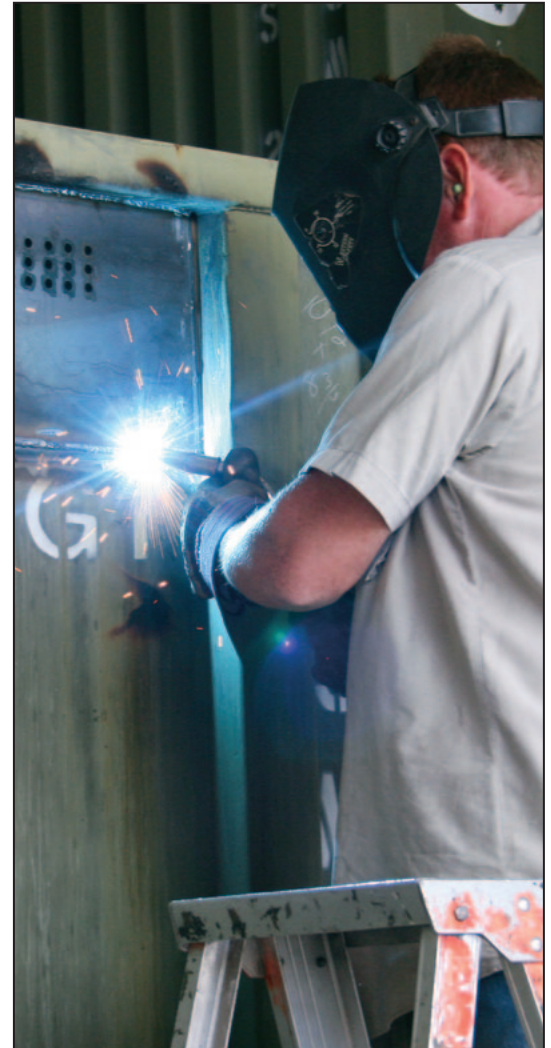
Container vent installation.
