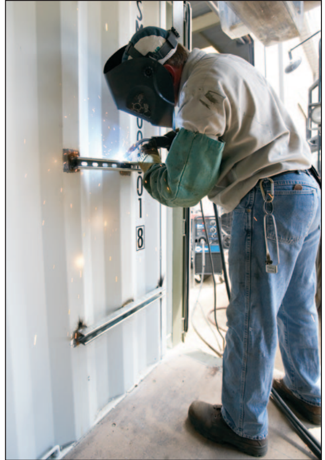
Specialized dry cargo container being modified for fire suppression system.
