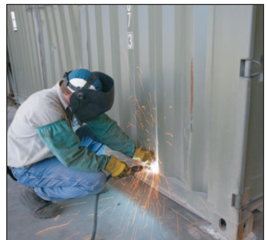
External fixture points being applied.
