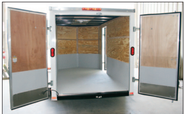
Polyurea coating applied to floor and interior sides of a small trailer.
