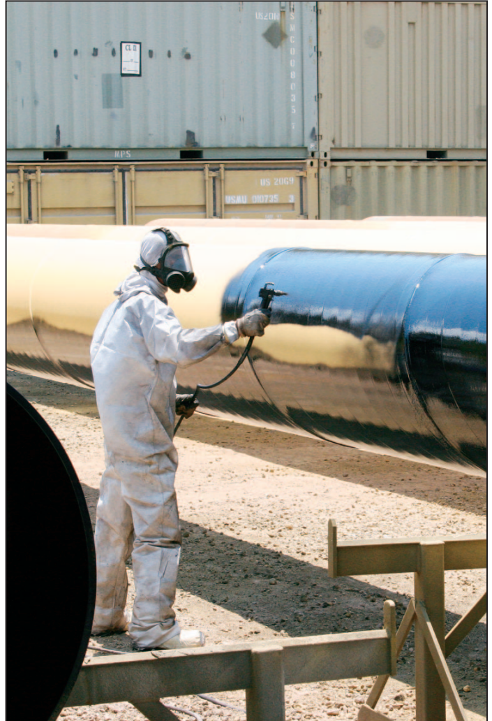
Coal Tar Epoxy being applied to 85' pylons.
